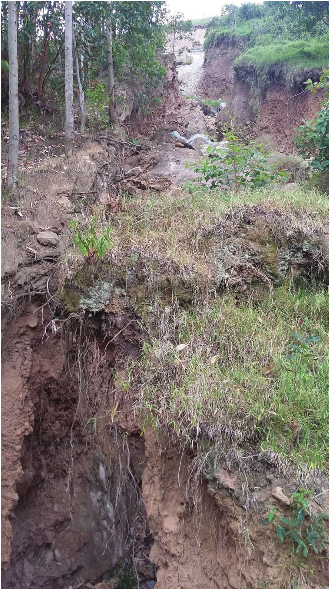
Plate 1: Landslides, rock falls and soil erosion hot spot in Kanaba Sub-county
